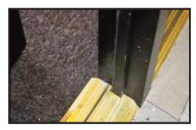
The base plate is attached within the thresholds to accept the mullion tube bottom.
