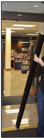
Having the mullion tube positioned between the single doors eliminate air flow while serving as an element barrier.
