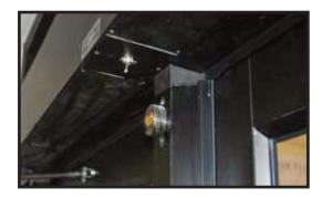
The locking mechanism is housed with in the mullion cavity to shield it from debris and unauthorized tampering.
